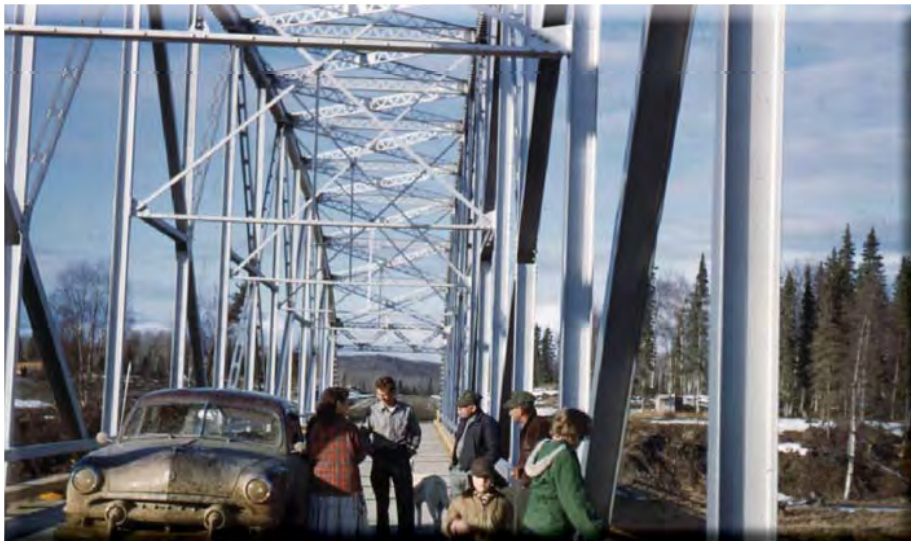
Kenai River Bridge, 1950s
