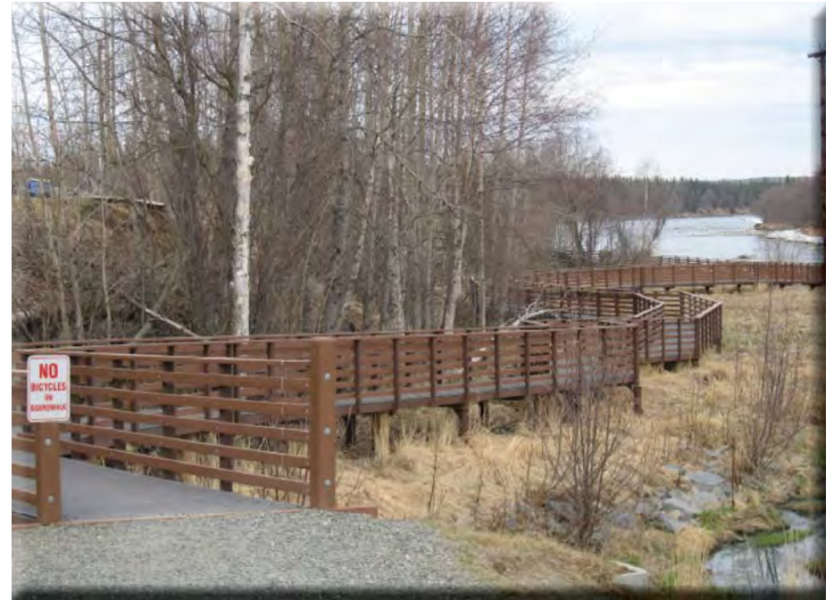
Kenai River boardwalk behind the Aspen Hotel
