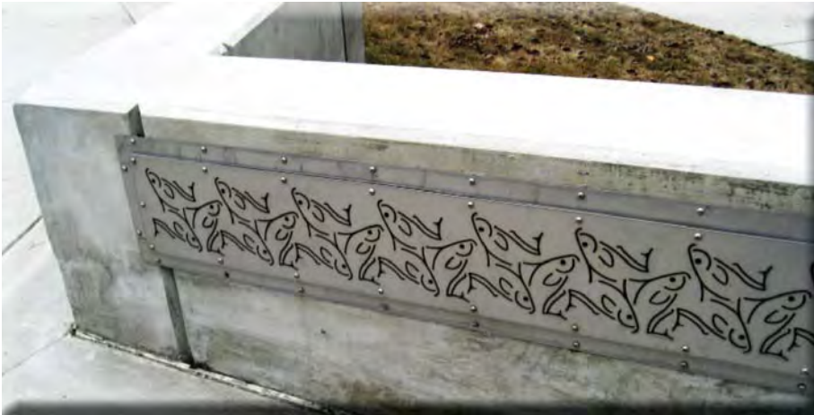
Local design features on a pedestrian bench along the Sterling Highway.
