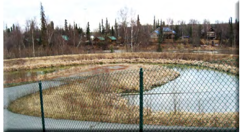
Storm water treatment system
