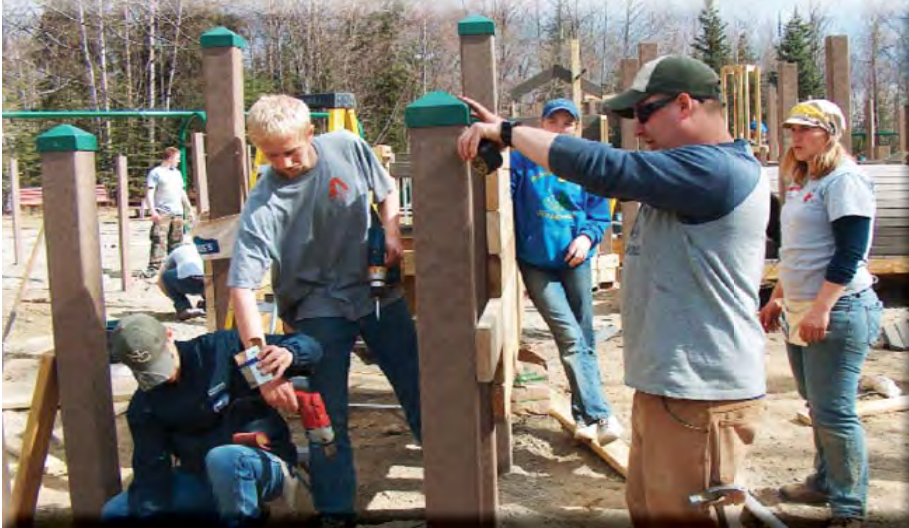
Members of the community volunteered to construct the new Soldotna Community Playground, located at Soldotna Creek Park.
