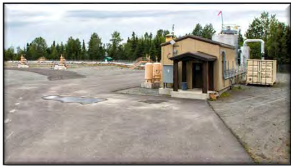
Gas Facility in Kenai
