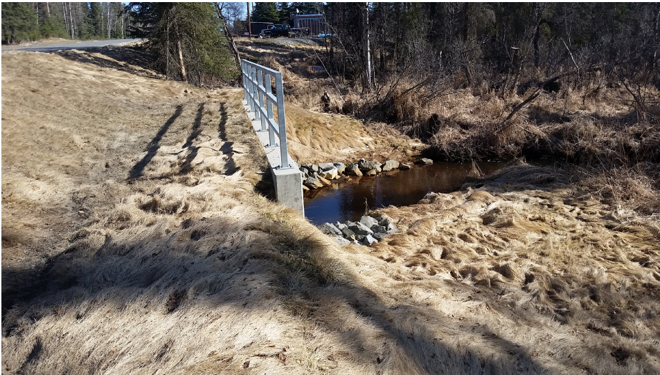
Completed bulkhead and culvert, downstream portion. Beaver Loop Road Culvert project 2016.
