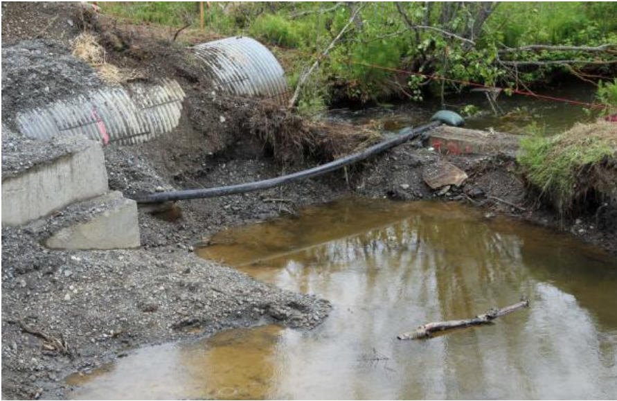
High levels of groundwater delayed the culvert replacement project on Beaver Loop Road that pushed the completion timeline back three weeks before the section of road could be reopened. (Credit: Peninsula Clarion)
