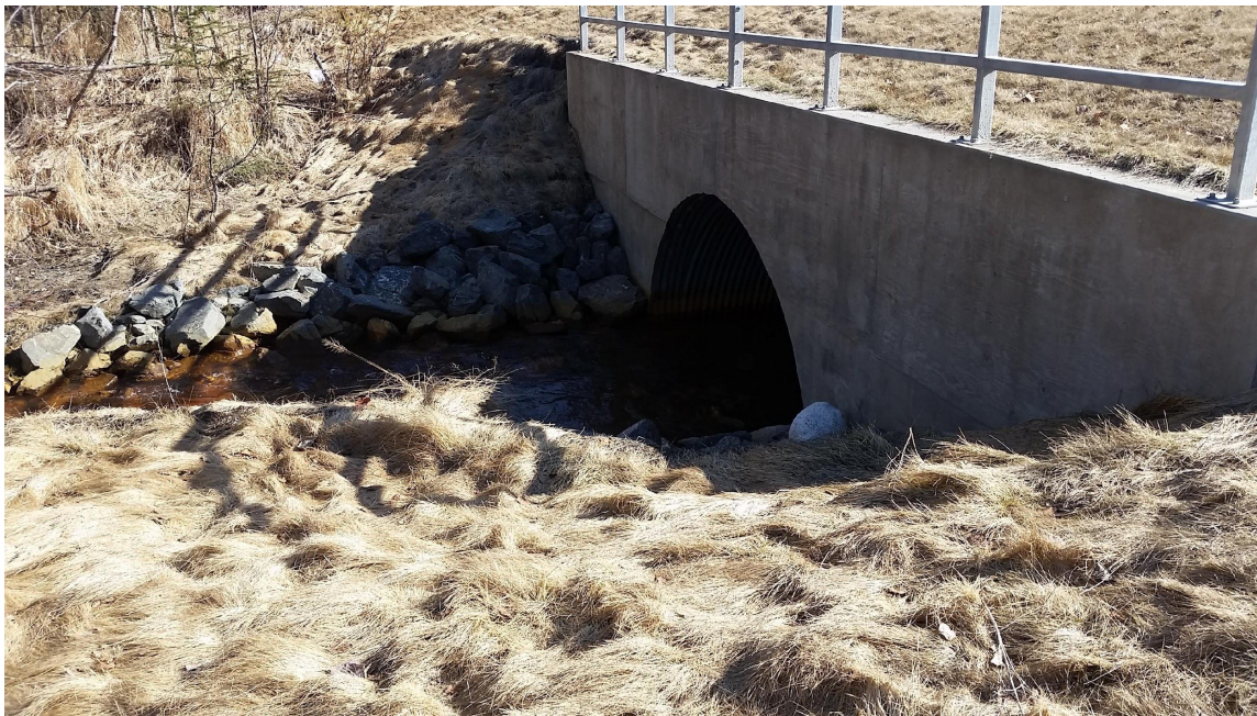
Completed bulkhead and culvert, upstream portion. Beaver Loop Road Culvert project 2016.
